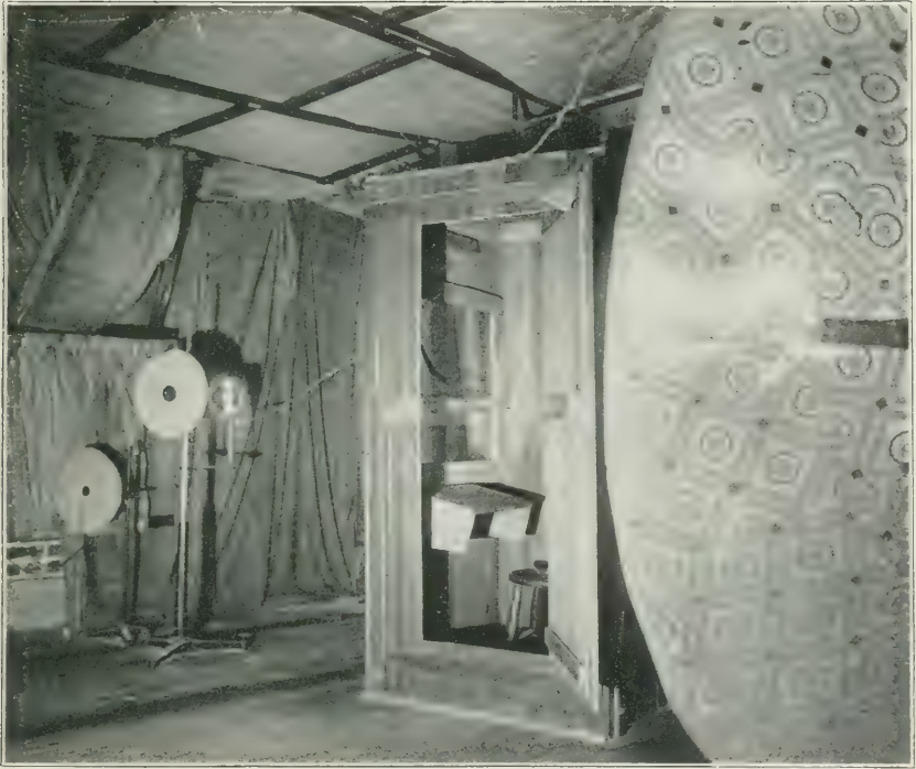
FIG. 12. VIEW OF TEST ROOM, SHOWING RAYLEIGH RESONATOR AND BOOTH FOR OBSERVER
